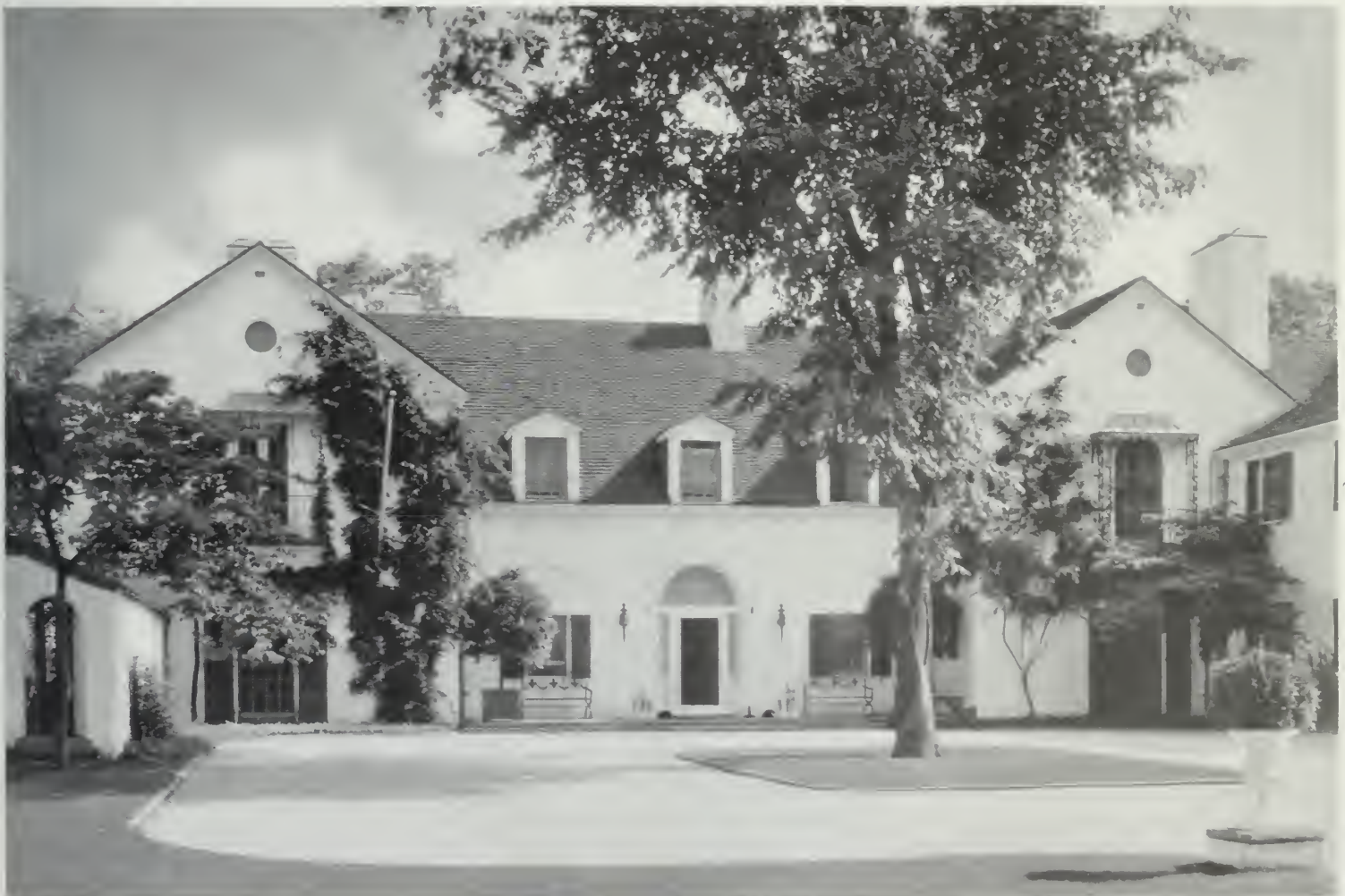
Finished and already covered with transplanted vine; the court yard and tree are shown in the background of the photograph of the model
